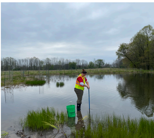
Wetland plug installation
