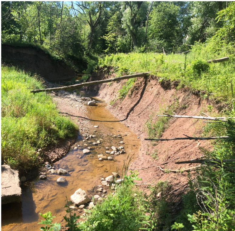
Extensive stream bank erosion is regrading habitat availability and water quality.
